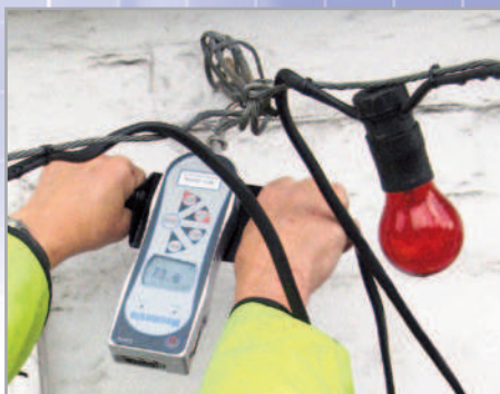
Pull test on anchorage points
